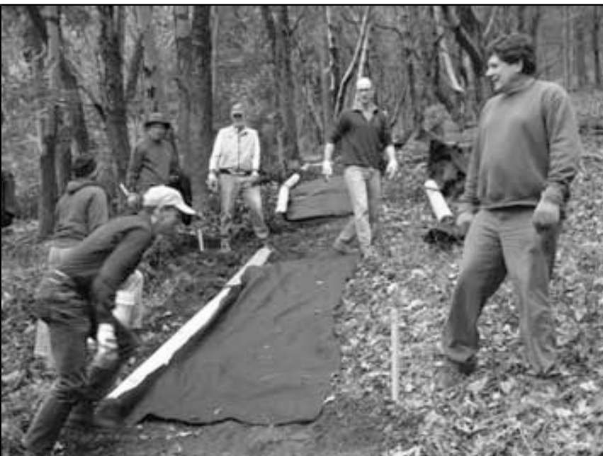
Hearts trail construction.
