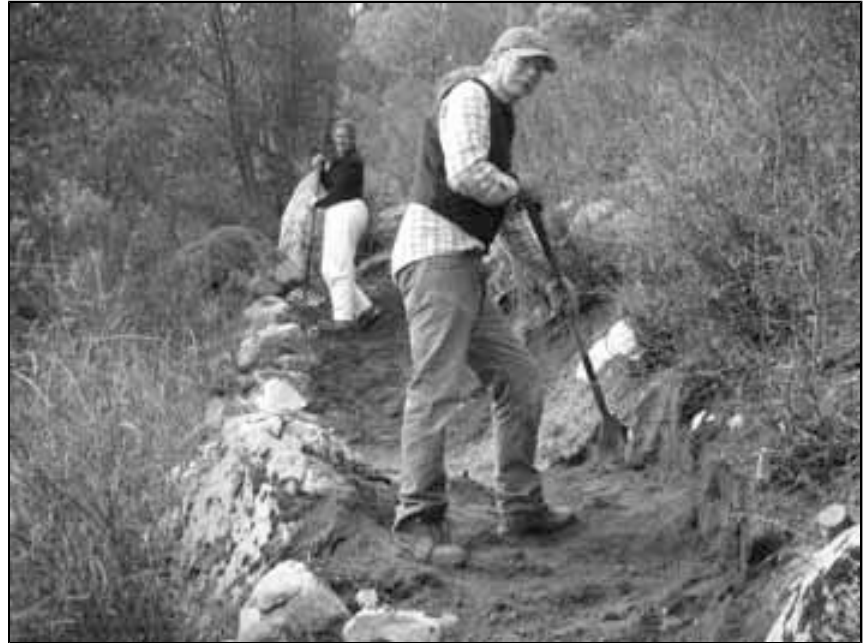
Looking Glass trail rehabilitation.
